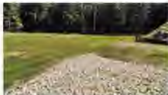
Photo 9 – Infiltration Basin, looking East Beachmont Subdivision – Old Orchard Beach, ME Taken by Steve Blais, 8/14/15
