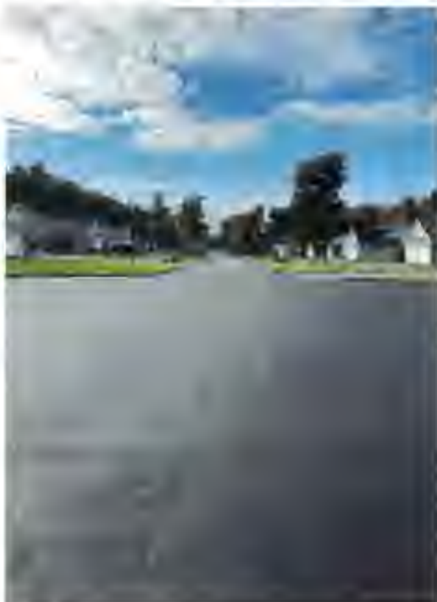
Photo 4: SE side of Dolphin Avenue paved, facing NW (Photo taken by Ron May Dated 10/2/2024)
