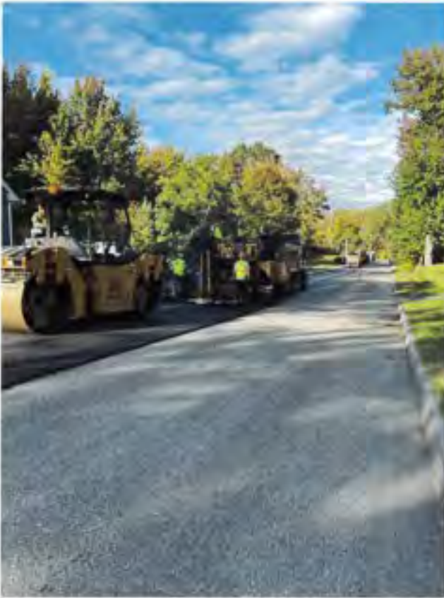
Photo 7: Paving and compacting Neptune Road, headed NE to its intersection with Portland Avenue (Photo taken by Ron May Dated 10/2/2024)
