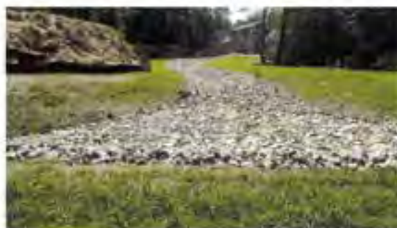
Photo 11 – Stone Level Spreader to Basin Beachmont Subdivision - Old Orchard Beach, ME Taken by Steve Blais, 8/14/15
