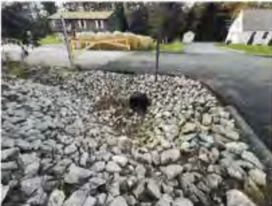
Cross culvert at Date Street intersection.
