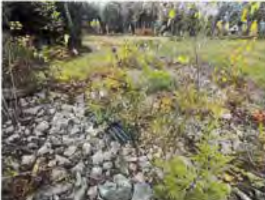
30" outlet to Infiltration Basin #1.
