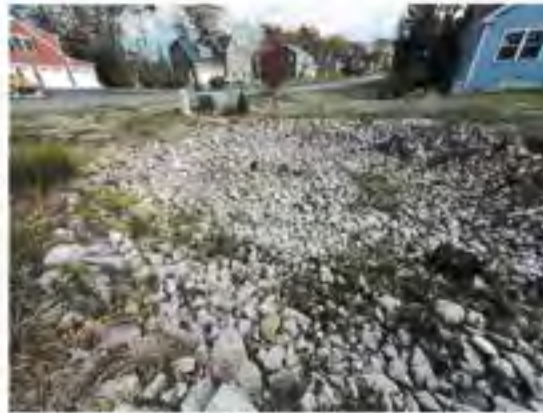
Forebay inlet on lot 32.
