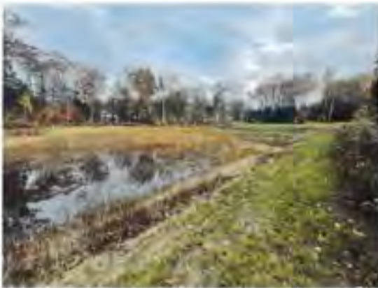
Infiltration Basin #1 looking east.
