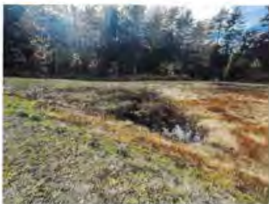
Infiltration Basin #1 sediment forebay.
