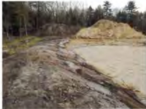
Photo 2 – Infiltration Basin, looking South Beachmont Subdivision - Old Orchard Beach, ME Taken by Steve Blais, 5/12/13
