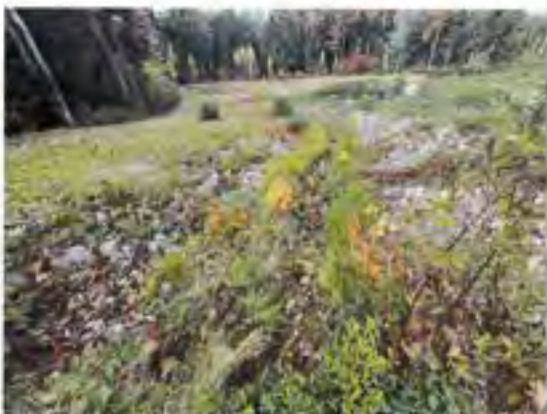
Armored swale inlet to Inf. Basin #1 looking downstream.
