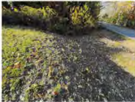
Embankment of Infiltration Basin #2 parallel to Portland Ave.
