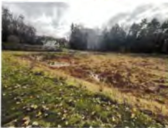
Infiltration Basin #1 looking west.
