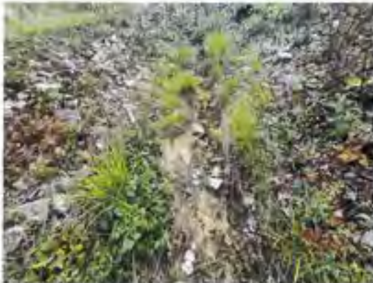
Erosion in armored swale to Infiltration Basin #1.
