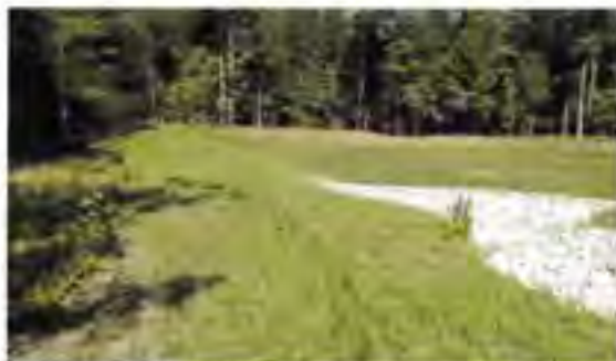
Photo 8 – Infiltration Basin, looking North Beachmont Subdivision - Old Orchard Beach, ME Taken by Steve Blais, 8/14/15
