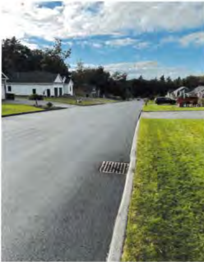
Photo 5: NW side of Dolphin Avenue paved, facing NW (Photo taken by Ron May Dated 10/2/2024)
