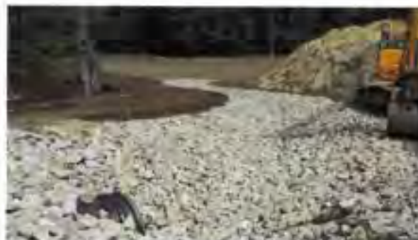
Photo 7 – HDPE Outlet to Infiltration Basin Beachmont Subdivision - Old Orchard Beach, ME Taken by David Alves, 7/8/15
