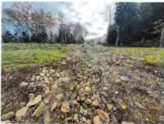
Armored swale inlet to Inf. Basin#1 looking upstream.
