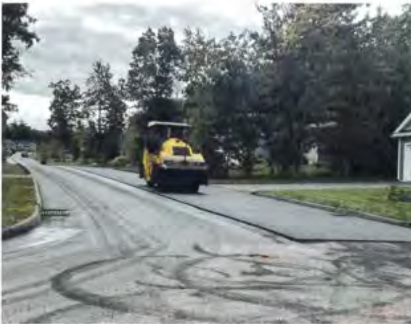
Photo 3: Roller compacting pavement near the intersection of Dolphin Avenue and Neptune Road, facing SE (Photo taken by Ron May Dated 10/2/2024)
