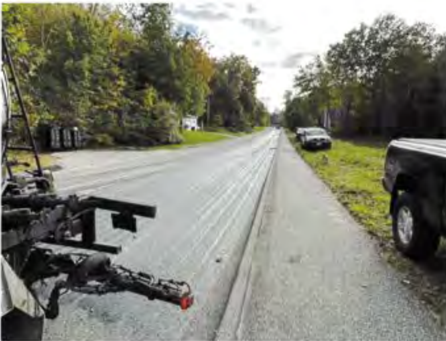
Photo 6: Tack coat on Neptune Road, facing SW (Photo taken by Ron May Dated 10/2/2024)
