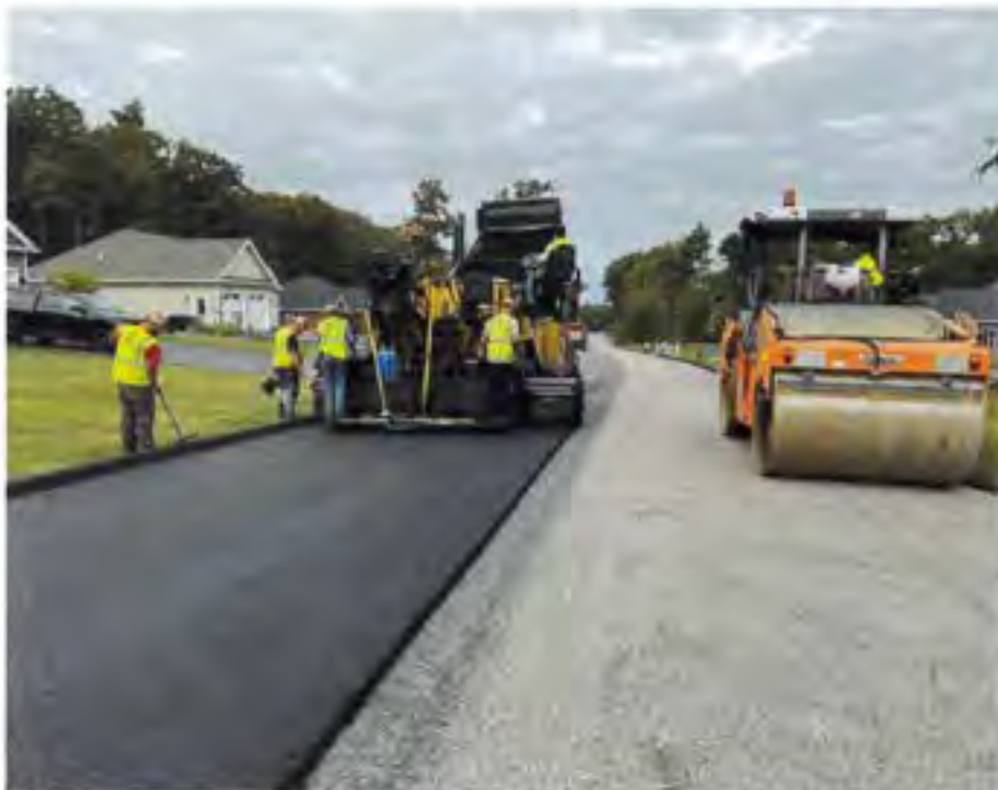
Photo 2: Paving headed NW on Dolphin Avenue toward its intersection with Neptune Road (Photo taken by Ron May Dated 10/2/2024)
