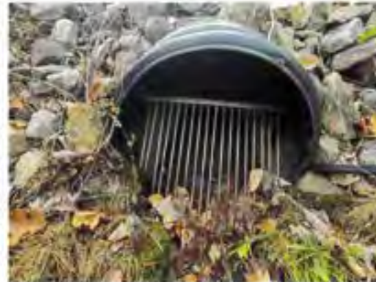
30" outlet to Infiltration Basin #1.
