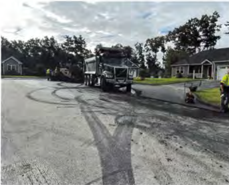
Photo 1: Start of paving on the SE end of Dolphin Avenue in the cul-de-sac (Photo taken by Ron May Dated 10/2/2024)
