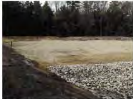
Photo 4 – Infiltration Basin, looking North Beachmont Subdivision - Old Orchard Beach, ME Taken by Steve Blais, 5/12/13
