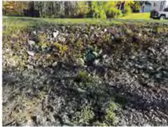
Inlet to Infiltration Basin #2.
