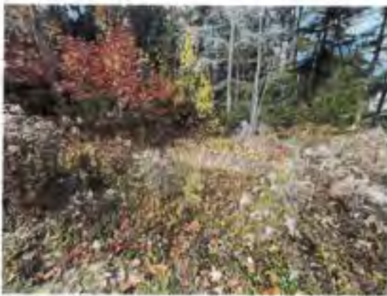
Eastern spillway of Infiltration Basin #1.
