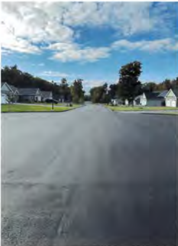
Photo 4: SE side of Dolphin Avenue paved, facing NW (Photo taken by Ron May Dated 10/2/2024)
