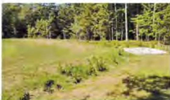
Photo 10 – Rip Rap Level Lip Spreader Beachmont Subdivision - Old Orchard Beach, ME Taken by Steve Blais, 8/14/15
