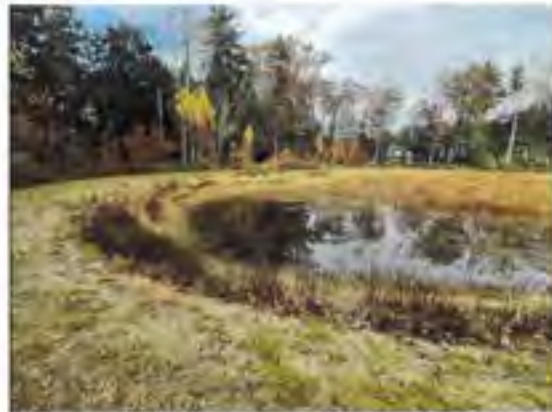
Infiltration Basin #1 looking northeast.
