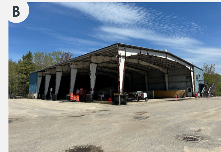
Salt & Sand Storage Building
