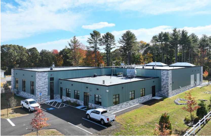
Operations entry and parking area.
