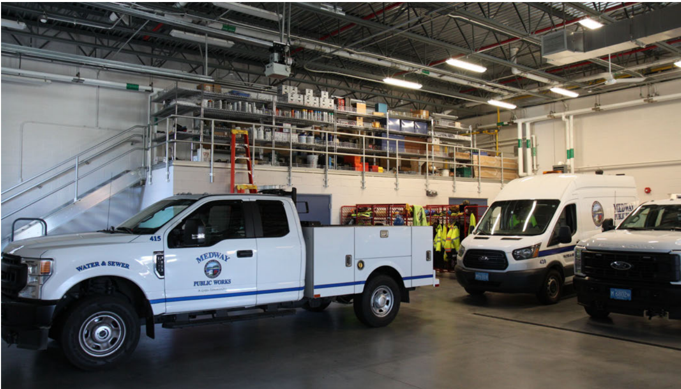
Garage and mezzanine storage area.
