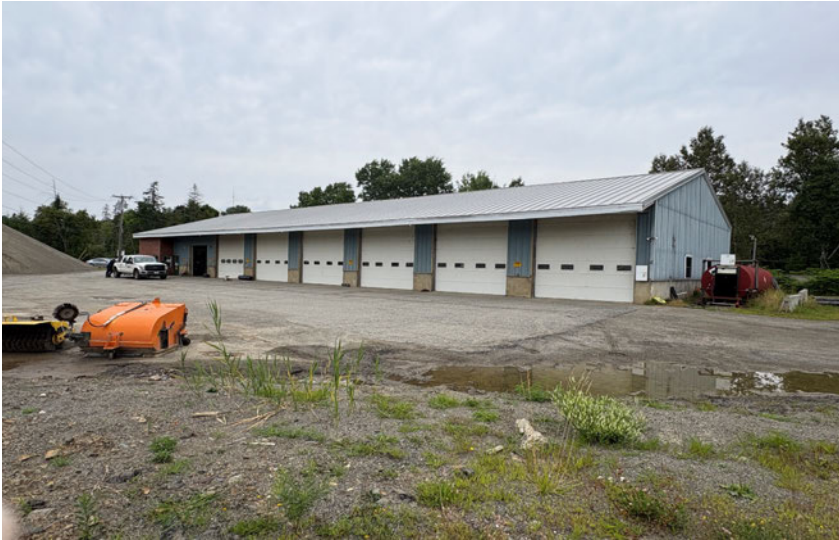
Town's existing highway department garage.
