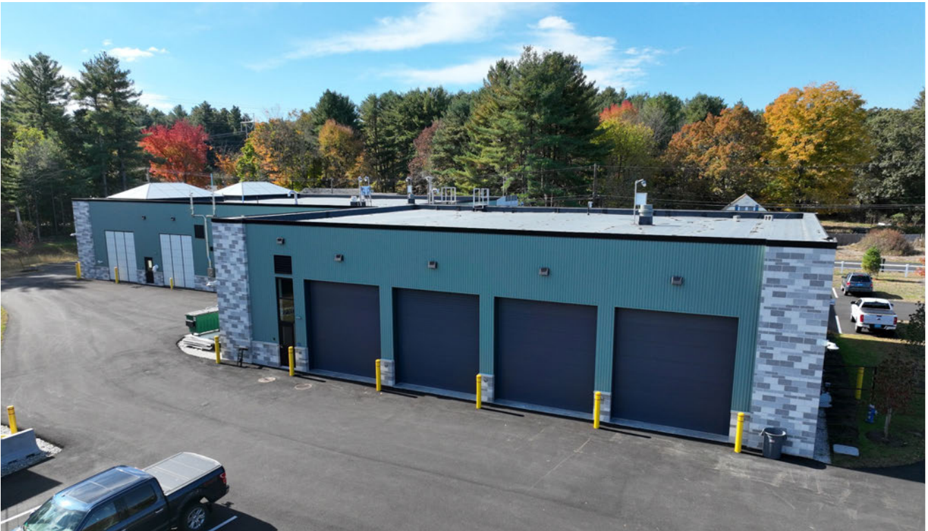
Garage and employee parking area.
