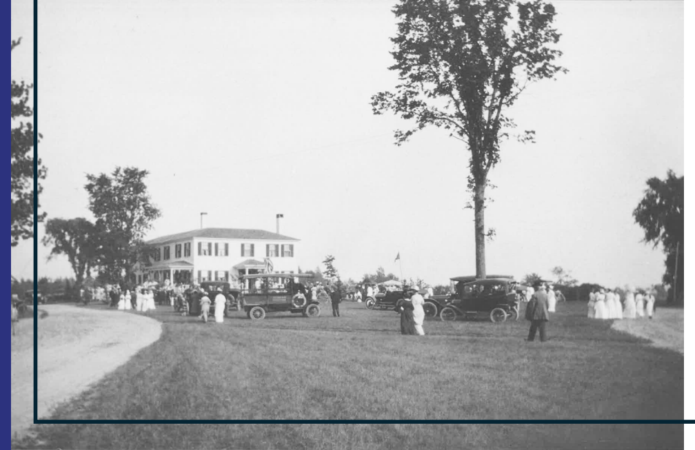
The RHR Smith & Company, CPAs office building pictured in 1914
