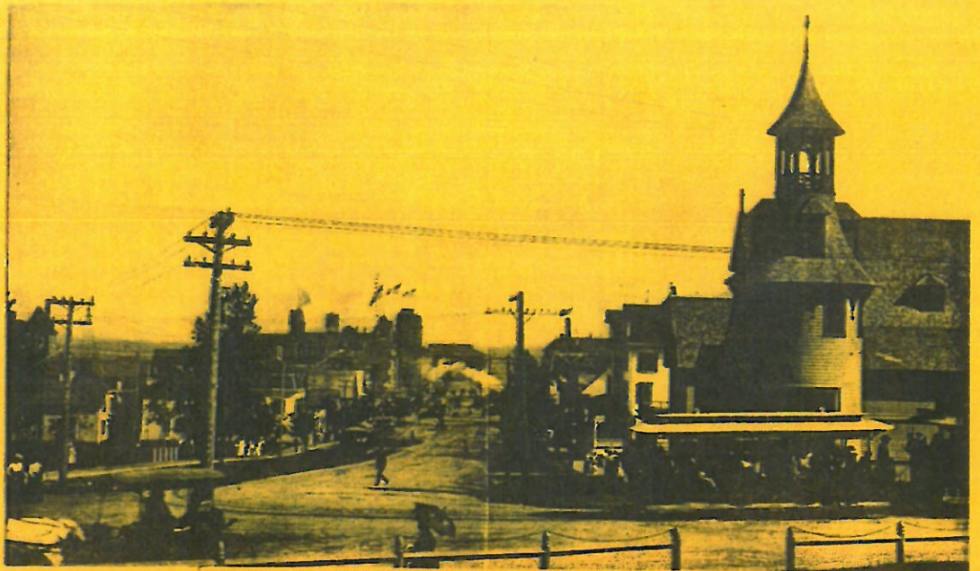
VIEW OF OLD ORCHARD STREET , 100 feet in width, looking towards the Ocean, showing line of trolley cars and steam railroad crossing; showing the relative location of the traction roads and distance from entrance to Sea Side Park to Station of the Boston & Maine R. R. The five white posts on extreme left mark the Park entrance from Main Street.
