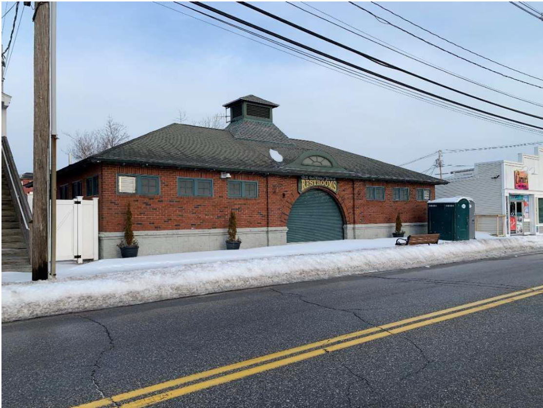
Photo 1: Building Front Exterior
