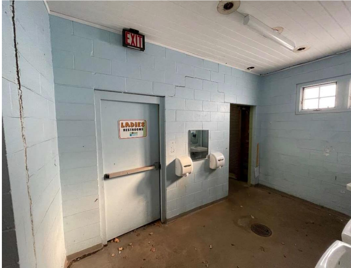
Photo 9: Building Interior, Women's Restroom
