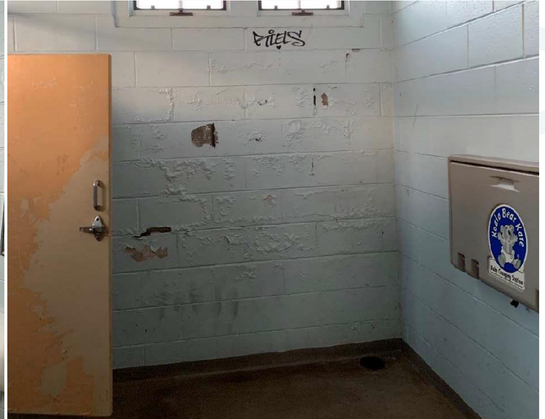
Photo 14: Building Interior, Men's Restroom
