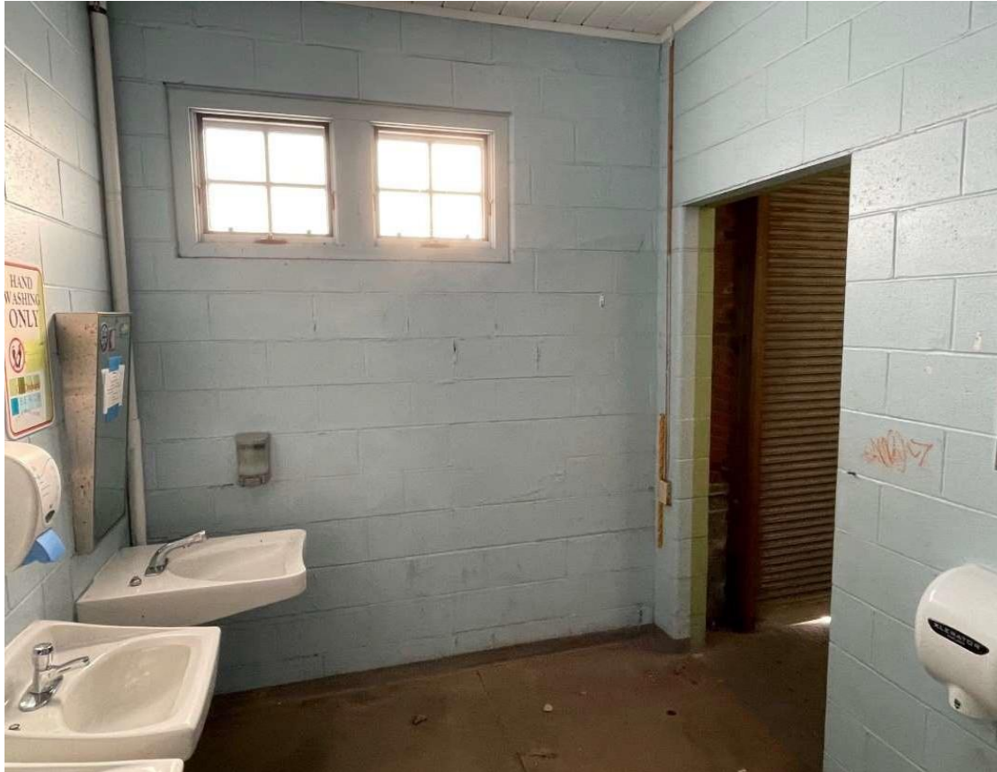
Photo 13: Building Interior, Men's Restroom
