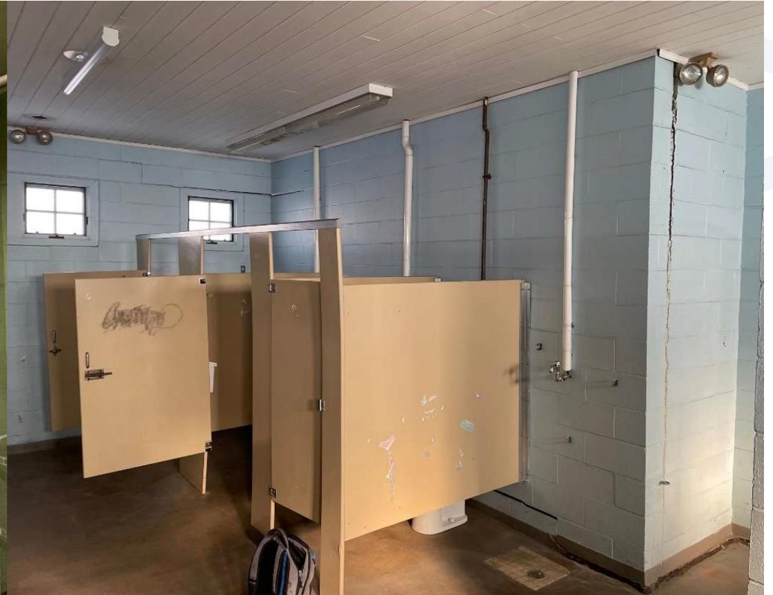
Photo 8: Building Interior, Women's Restroom
