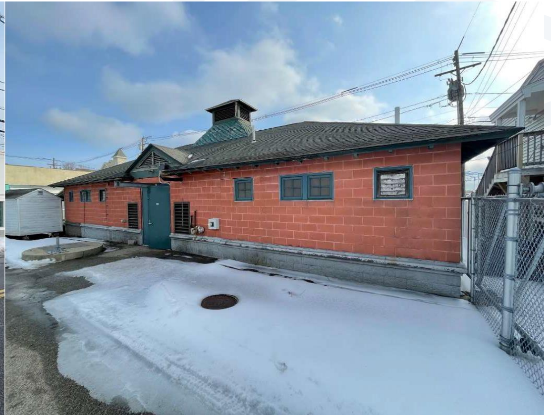
Photo 2: Building Rear Exterior
