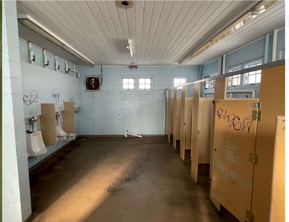
Photo 12: Building Interior, Men's Restroom
