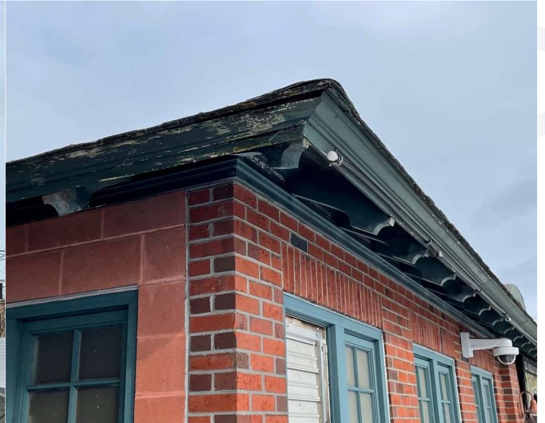
Photo 6: Building Rafter Tails and Trim
