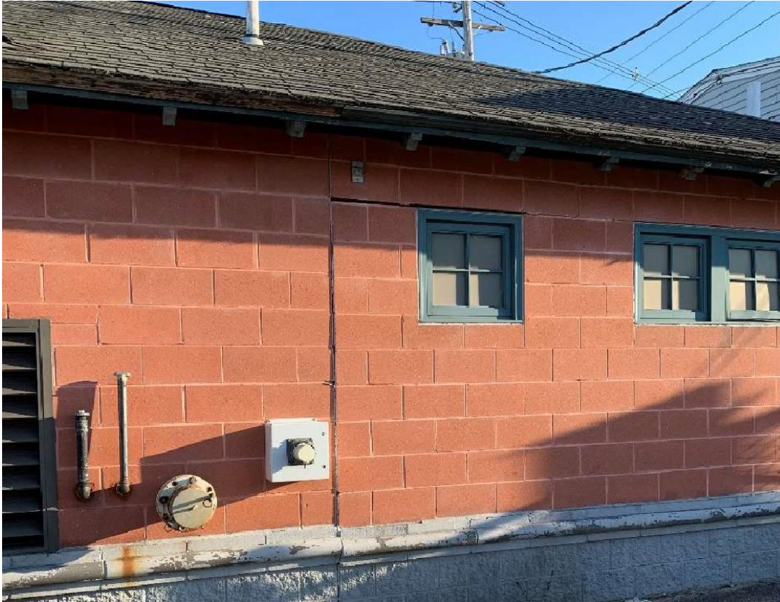
Photo 2: Building Rear Exterior
