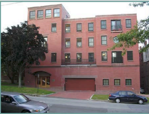
Casco Terrace 2004 27 apartments
