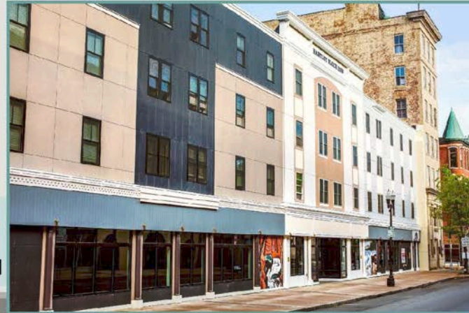
The Hartley Block , Lewiston 2019 63 apartments / 4000 sf retail
