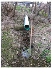
This outfall, though in poor condition because it is cantilevered, provides a good opportunity for a clean catch of its discharge.
