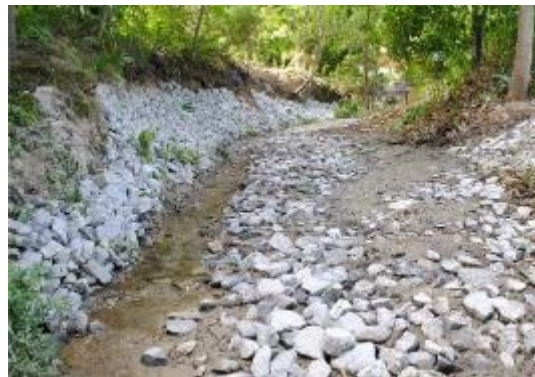
Examples of findings from the RGA, bank armoring at Upper Bear Brook. PHOTO CREDIT: John Field (see Field 2015)
